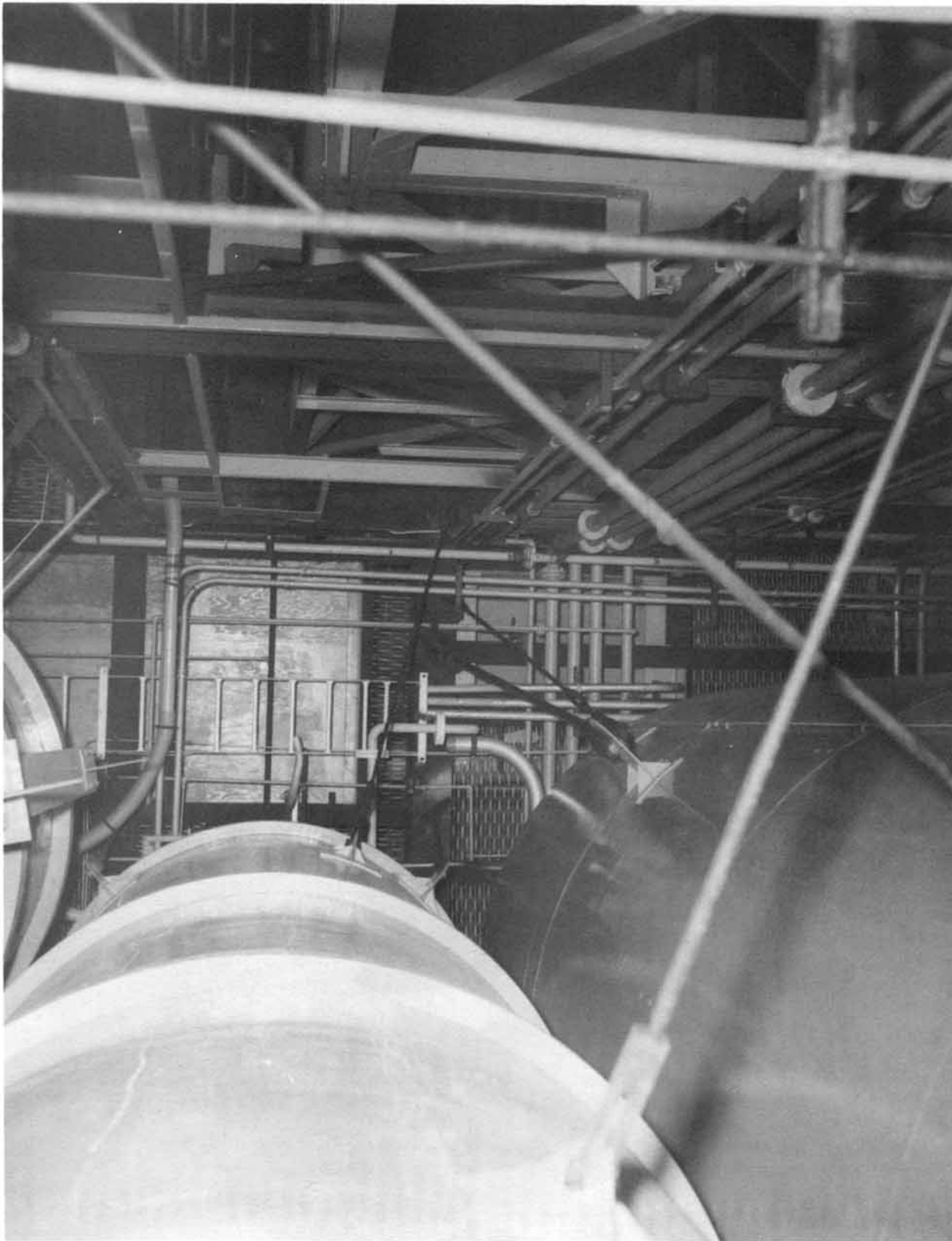
Looking up to Level 7 from near Column K (Neg. No. 68082A dated 4-27-61).
