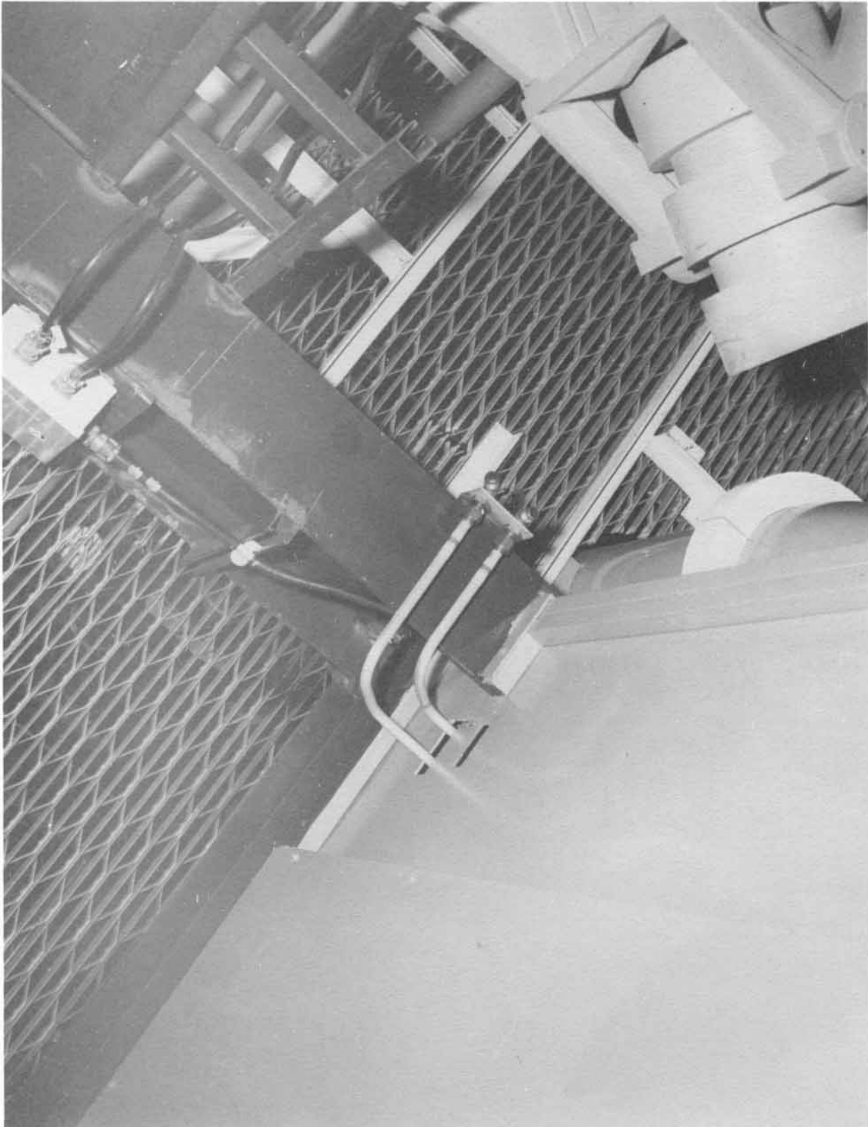
Hydraulic tubes to crib lock at Column D (Neg. No. 64932A dated 2-27-61).
