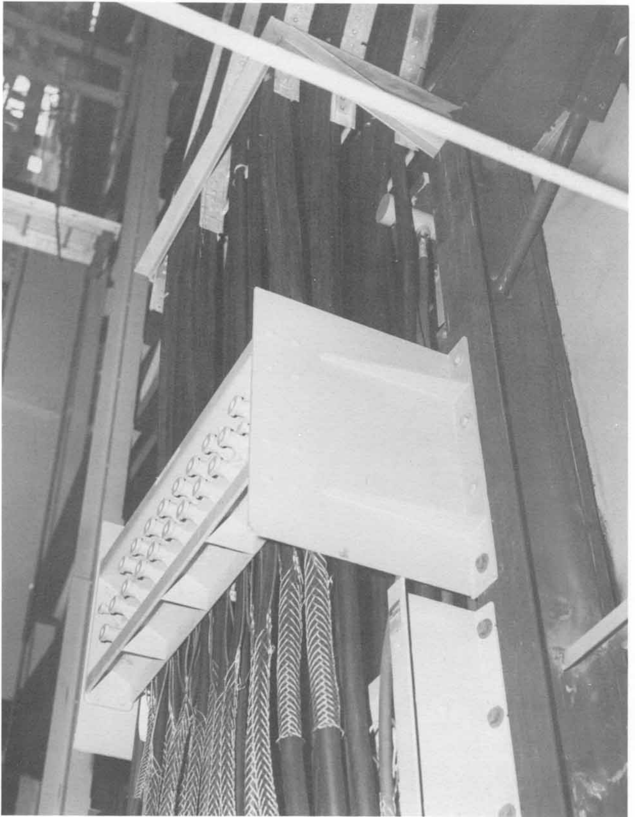
Cable loop bracket (Neg. No. 67330A dated 4-14-61).
